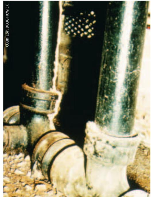
*Mud shelter tubes over subfloor piping are signs of termite activity.*
