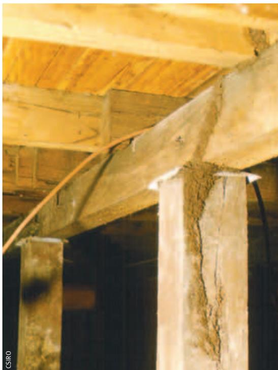
*Metal termite shields, also called ant caps, don't prevent termite activity, but it's easier to spot the tubes as they cross the cap.*
