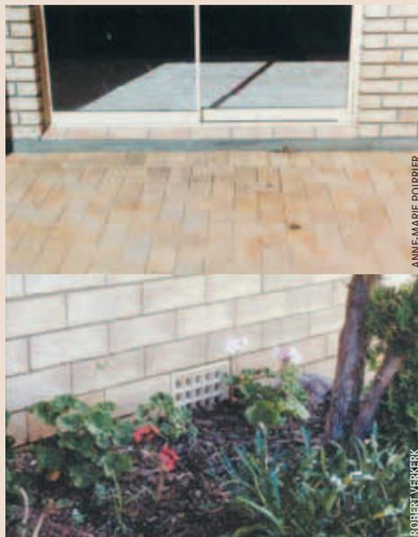
*An exposed concrete slab, like the one in the top photo, acts as a physical barrier that will bring termite activity into the open. If it’s covered with shrubs and plants, as in the photo below, termites can gain concealed access to structural timbers.*
